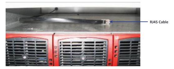
Connect the RJ45 cable placed on the top of the inverter shelf (when top cabling cabinet) on the first display's top plug. Make sure that this RJ45 comes from the same shelf where the T2S is installed.
